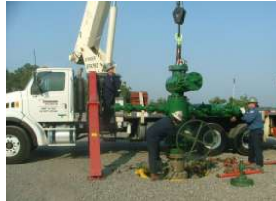
Installation of Seaboard™ frac tree
