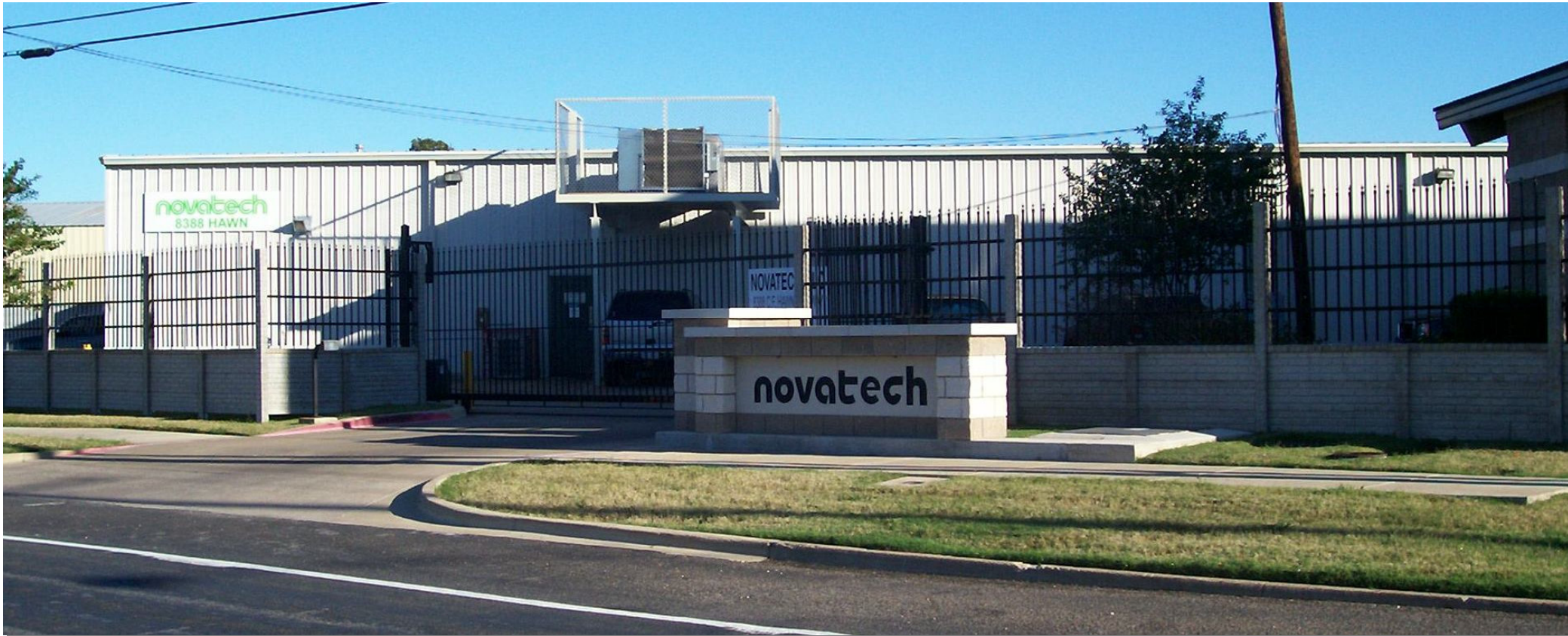
Novatech manufacturing facility and head office, Near Dallas, Texas
